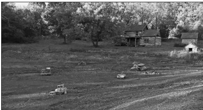
Completed fish habitats in Small Pond basin
