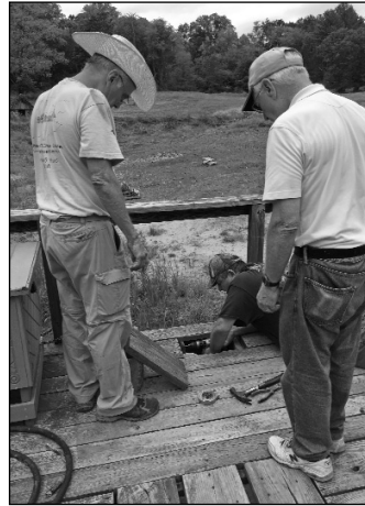
Installing pipe for locating drain valve
